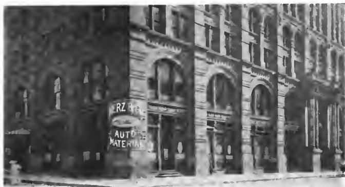
New Headquarters of Herz & Company, New York City.
